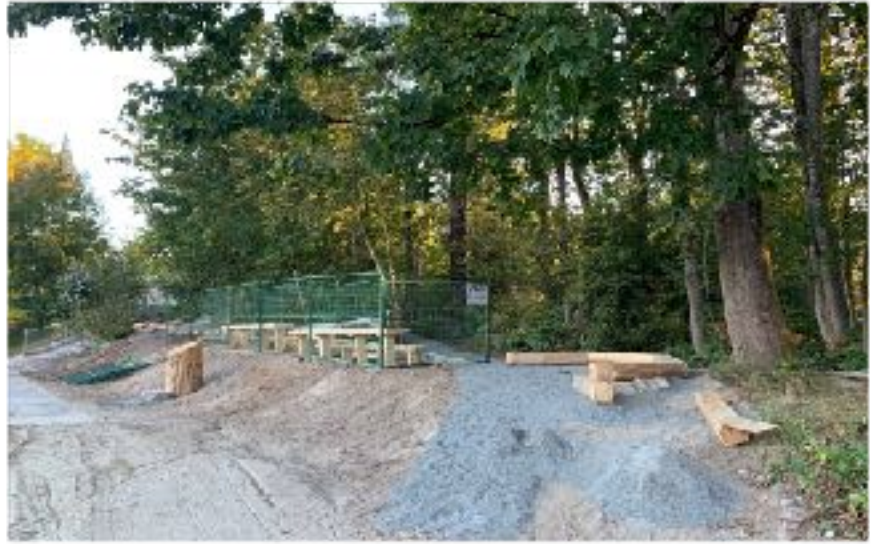
Construction of the new natural play and learning space.
